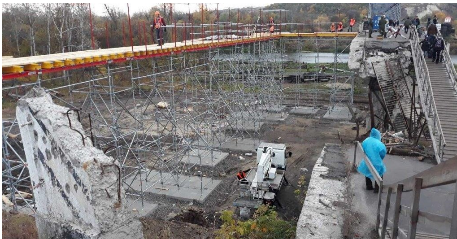
Ongoing construction of a bypass bridge at Stanytsia Luhanska (Jonas Leissner/OSCE)
