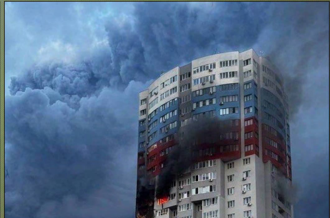
May 14 . An apartment building damaged as a result of a massive UAV strike on the city of Ryazan, Ryazan region. Four civilians were killed , including one child , and 28 were injured , four of whom were children.
