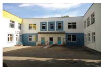
Thermal insulation and double-glazing in kindergarten № 45 in Grodno»
