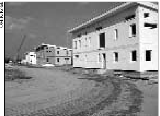
The South East European University in Tetovo, under construction in June 2001
