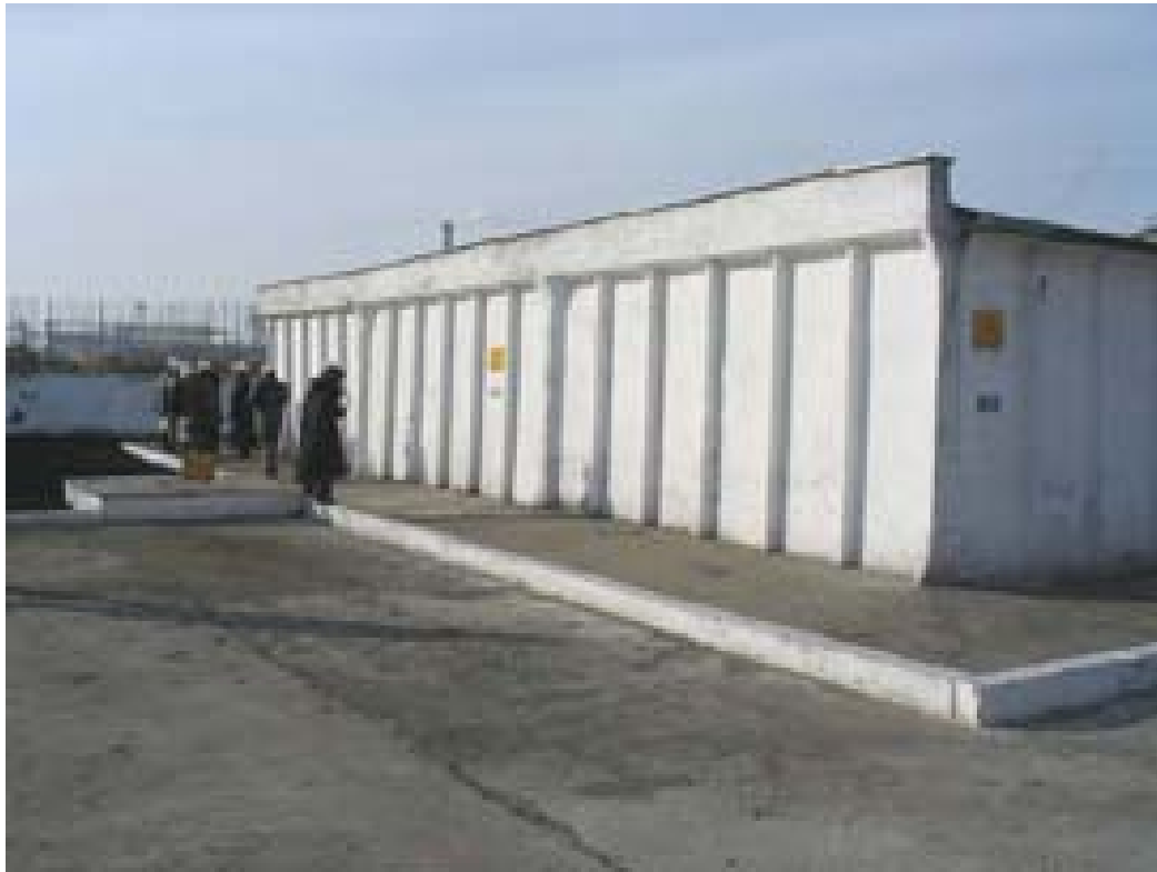
Figure 3: Side view of the contaminated dust storage facility
