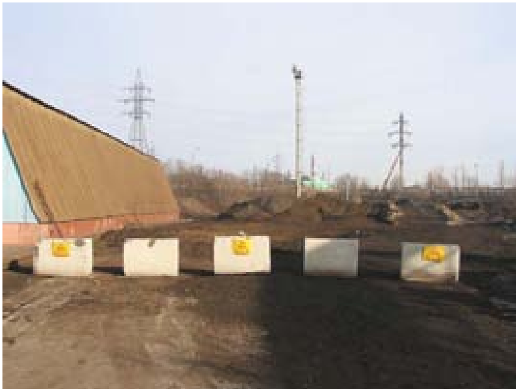
Figure 8: Entrance of the open-air dust storage site and the storage building (left) for contaminated steel product
