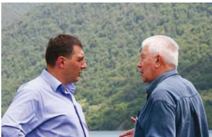
Alan Gabaraev, director of Energy Resources, based in Tskhinvali (left), and Konstantin Predein, a hydro-mechanical engineer with Georgia Water Project, based in Tbilisi (right), on the crest of the Zonkari Dam. The EU-funded OSCE project to restore the dam will improve the safety of the population and involves engineers from both Tbilisi and Tskhinvali. (OSCE/Emmanuel Anquetil)
