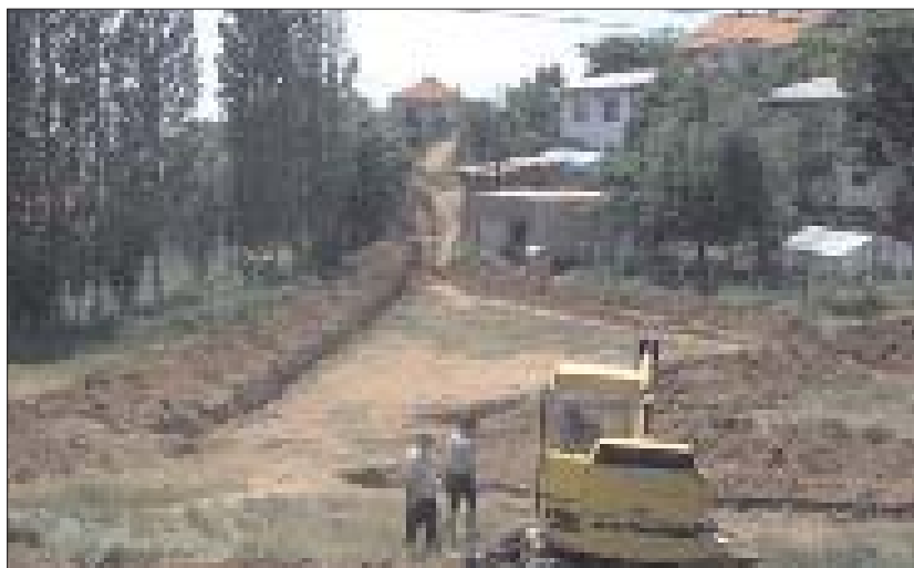
Digging channels for the water system
