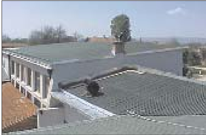
The new school roof in Vrbovac/Vrboc
