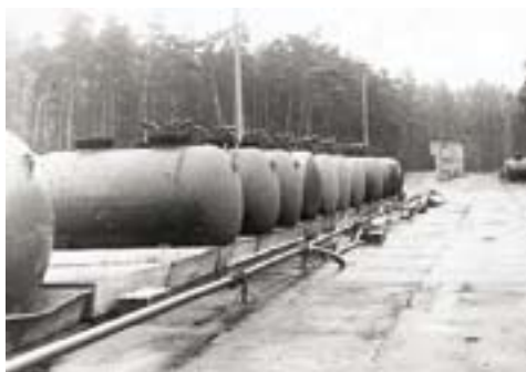
Fig. 5: Examples of safe melange storage
