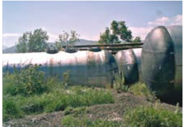
Fig. 2: Melange storage site in Armenia
