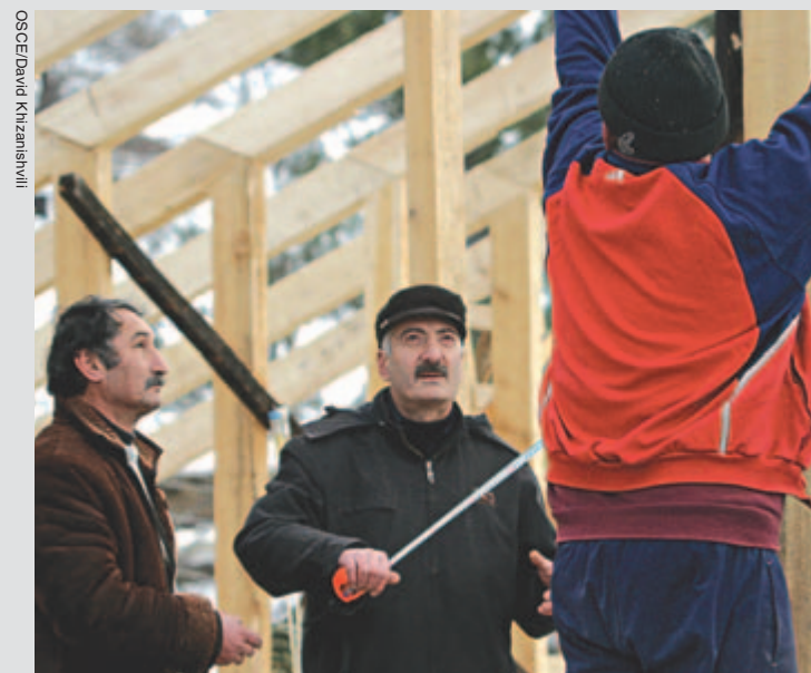
Working on urgently-needed renovations of a school in the north of the zone of the Georgian-Ossetian conflict. Bessarion is a local Ossetian contractor who won the tender to renovate this school in Dzari, one of the many rehabilitation projects earmarked by the OSCE-led Economic Rehabilitation Programme. For this renovation, Bessarion employed a workforce of builders from both Georgian and Ossetian communities, as well as three Ossetians from village of Dzari itself.
