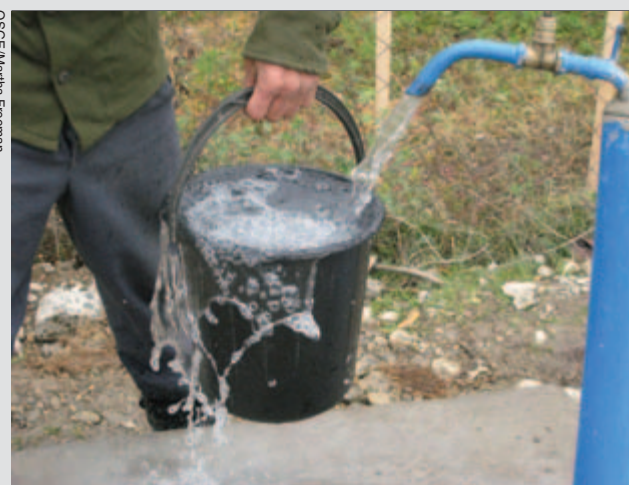
Drinking water on tap for the first time in some villages in the zone of conflict. Ksuisi, Disevi, Khelchua and Gugutiantkari villages now have drinking water after the OSCE-led Economic Rehabilitation Programme constructed 18 taps and 11km of pipes linking them to the local water supply.
