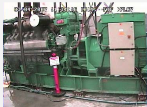
The diesel generator used in the Aurora Generator Test beginning to smoke
