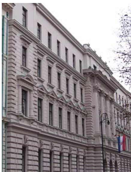
Zagreb County Court
