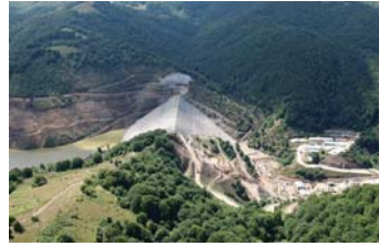
Dam construction in Macedonia
