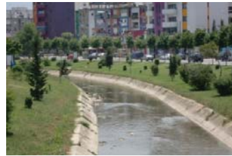
Sewerage system improvement in Albania
