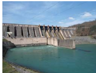
Rehabilitation of Hydro Power Plant in Bajina Basta
