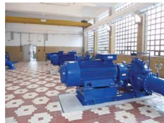
Water distribution pumps in Belgrade
