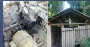
Small hydropower plants in Pingun, Rasht Valley, 19 September 2013
