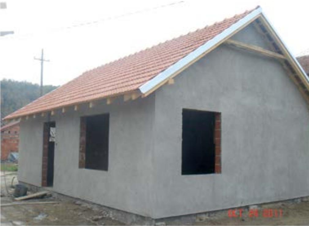
Photo 30: Completed rendering on a new house in Kraljevo after the earthquake
