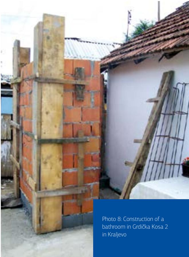
Photo 8: Construction of a bathroom in Grdička Kosa 2 in Kraljevo
