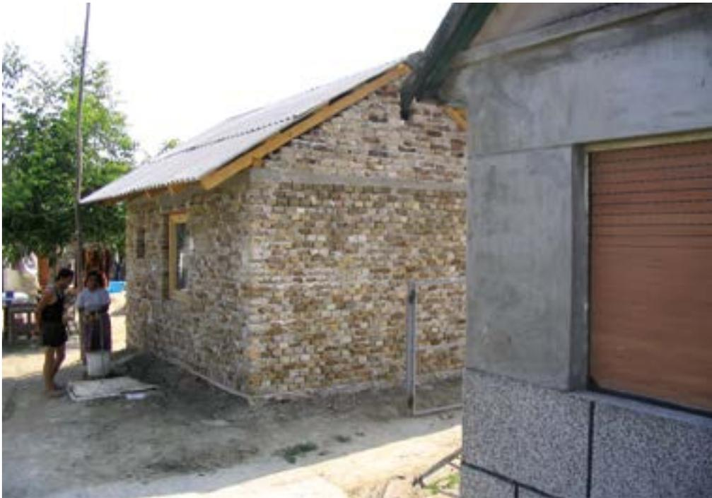
Photo 2: A new house built using recycled bricks in Apatin
