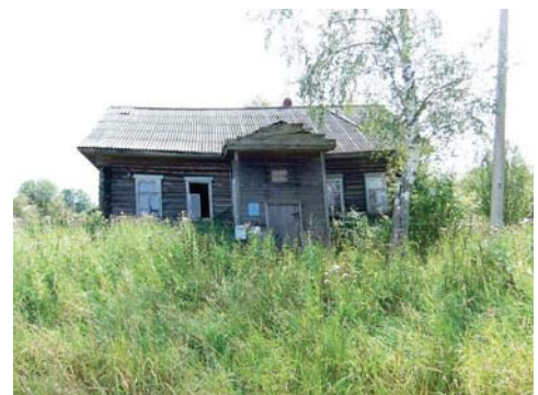
Abandoned rural building, Russia (Wikipedia)
