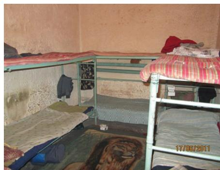
The observers found that in the TDFs of Djail, Tyup, Uzgen and Kadamzhai District IABs, the cells are in poor condition and need urgent repair. Humidity in these cells is very high, which is why mold fungus appeared on the walls.
