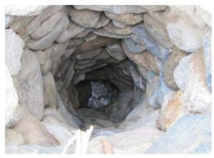
There are outdated irrigation and drinking water systems in Alvank and Shvanidzor communities of Meghri, underground tunnels with a length of around 1500 meters in Alvank and around 1200 meters in Shvanidzor. They consist of water tunnels and wells which are provided for maintenance of the system. Water flows into the system from mountain springs. The local population uses that water for both irrigation and drinking purposes. The irrigation
