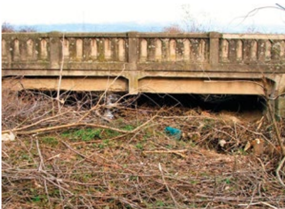
Figure 4: A typical example of the congestion of bridge opening that impedes the flow of water
