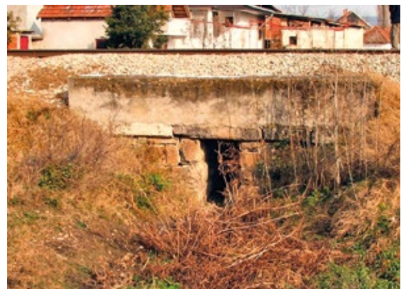
Figure 5: Characteristic method of increasing the transportation capacity of railway culvert by reducing the opening
