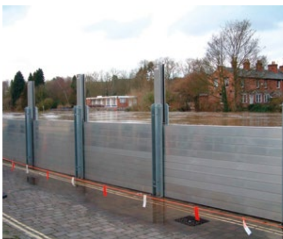
Figure 30: Demountable barrier in use
