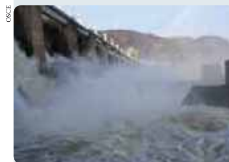
Kladovo power station, photographed during an outreach visit to eastern Serbia by the Head of Mission and his staff.
