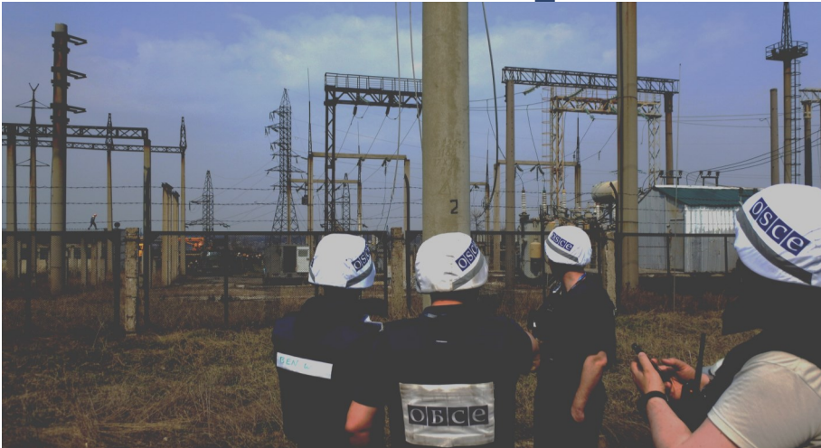
OSCE SMM monitors are facilitating and monitoring adherence to ceasefire to enable de-mining and repair at power lines and the substation near the Donetsk water filtration station Between Avdiivka and Yasynuvata, 4 April 2017 (OSCE/Edward Crowther)
