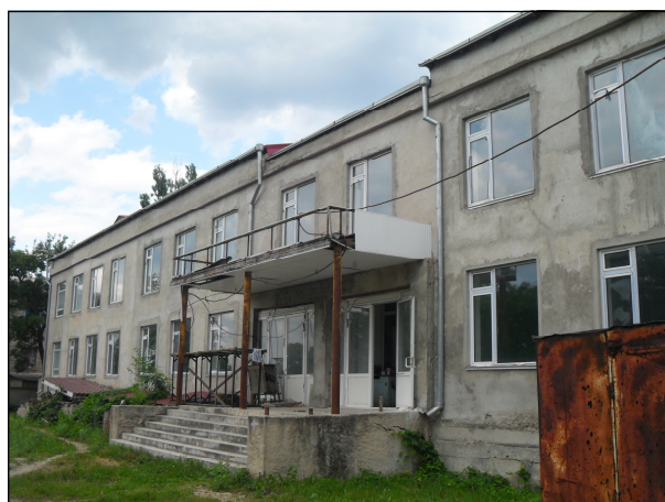
One of the buildings at 14 Gagarin Street in Ribnita, constructed at the expense of the Moldovan Ministry of Education
