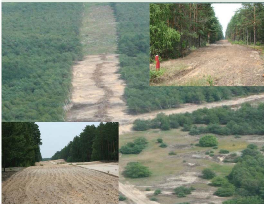
40 and 12 meters fire brake in plantations of the first category of natural fire risk
